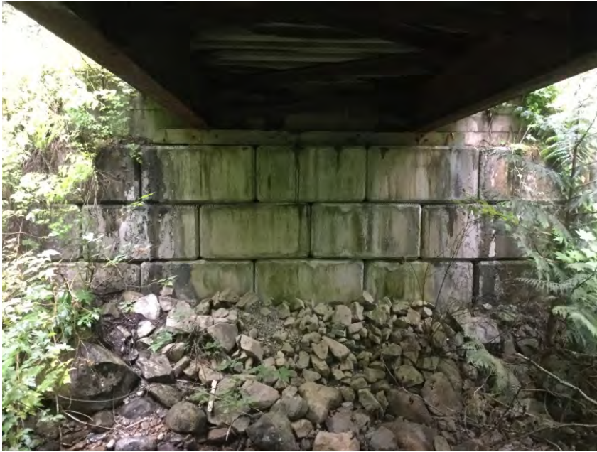
Left Bank Abutment when facing downstream
