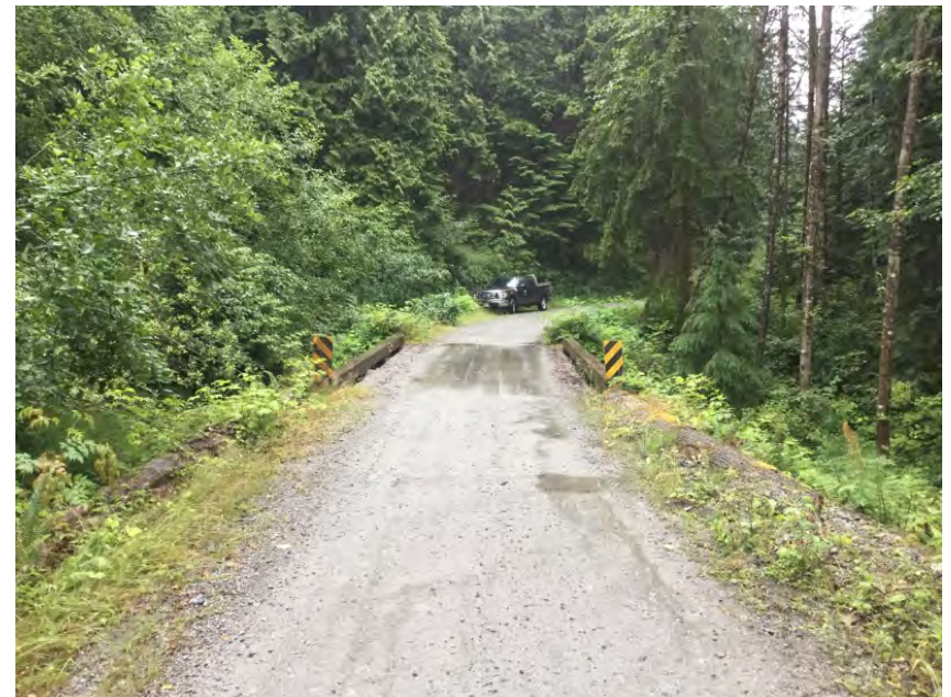
Approach from Right Bank when facing downstream
