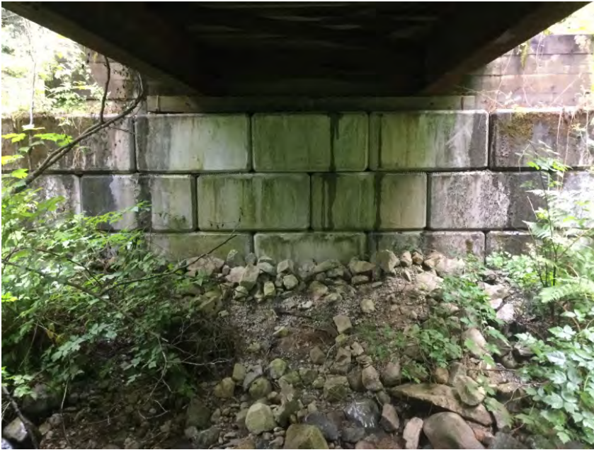
Right Bank Abutment when facing downstream
